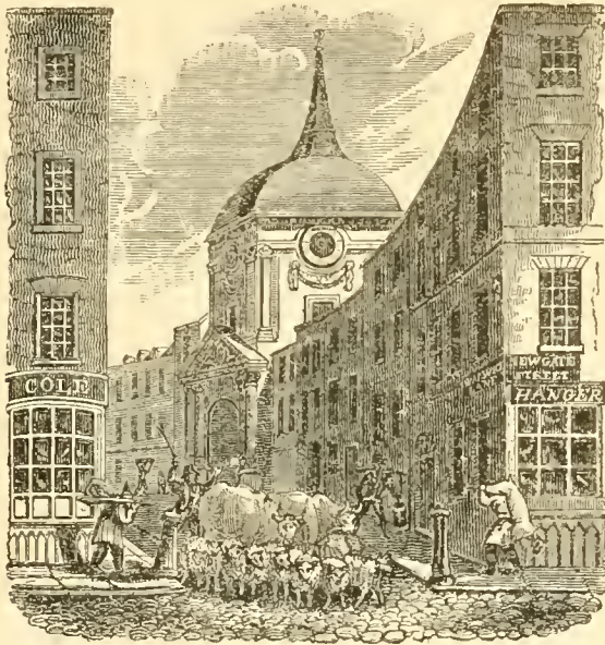
OLD COLLEGE OF PHYSICIANS, WARWICK LANE, NEAR NEWOATE.
